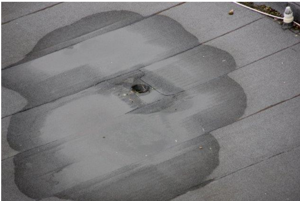
▲ F.02 Poor detailing preventing water from draining into gully
