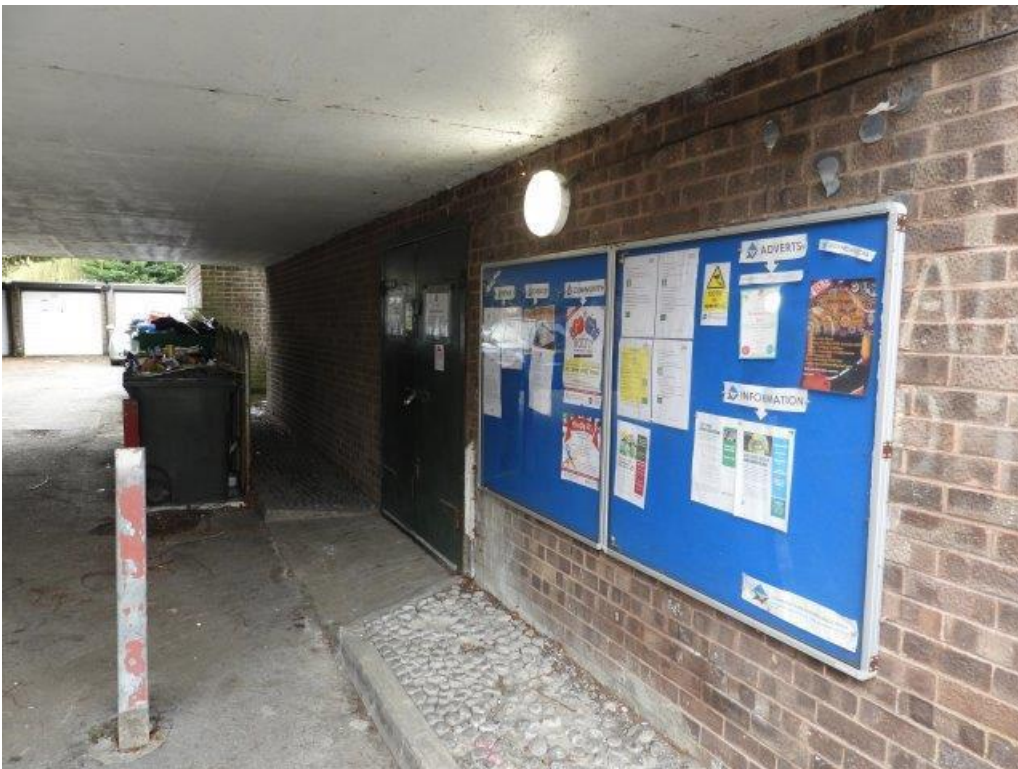
▲ F.46 Noticeboard showing confusing and incorrect information
