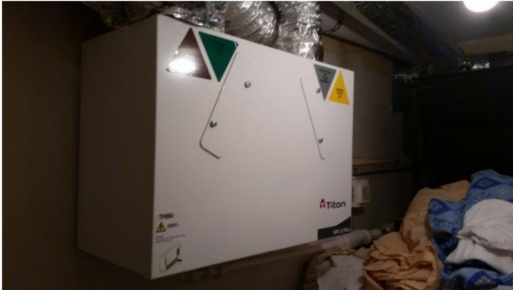
▲ F.31 HRV systems poor performance
