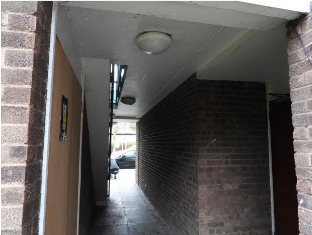
▲ F.27 Stair soffits and ceilings requiring decorations
