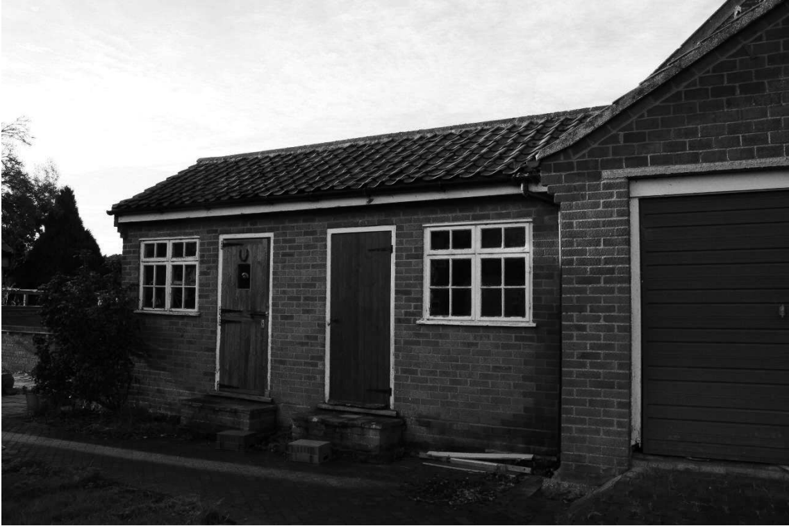
5. Rear store extension to garage
