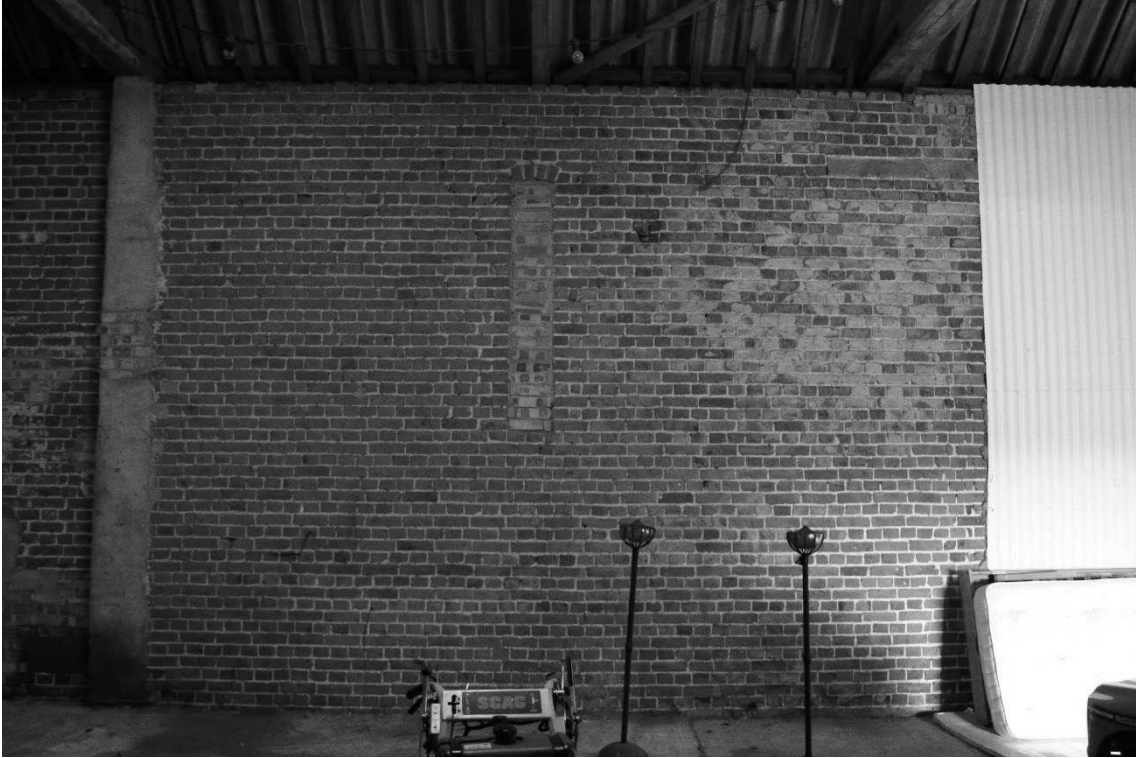
9. Typical internal view of front wall showing infilled door opening
