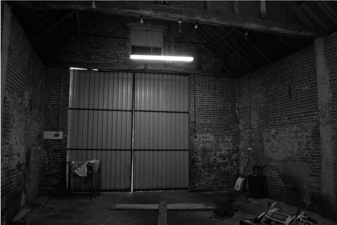
8. Internal view of right hand end wall
