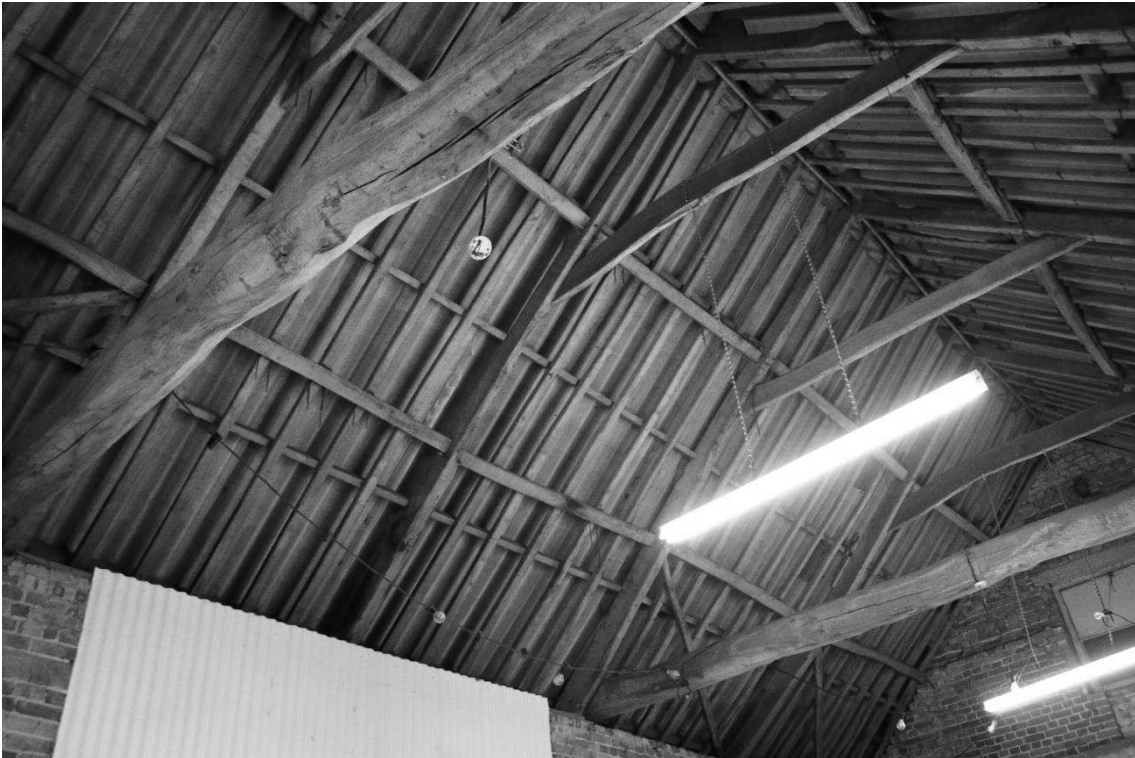
7. General view of barn roof structure
