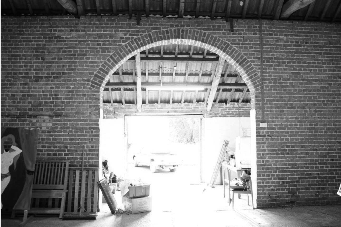
12. Archway to rear elevation through to offshoot
