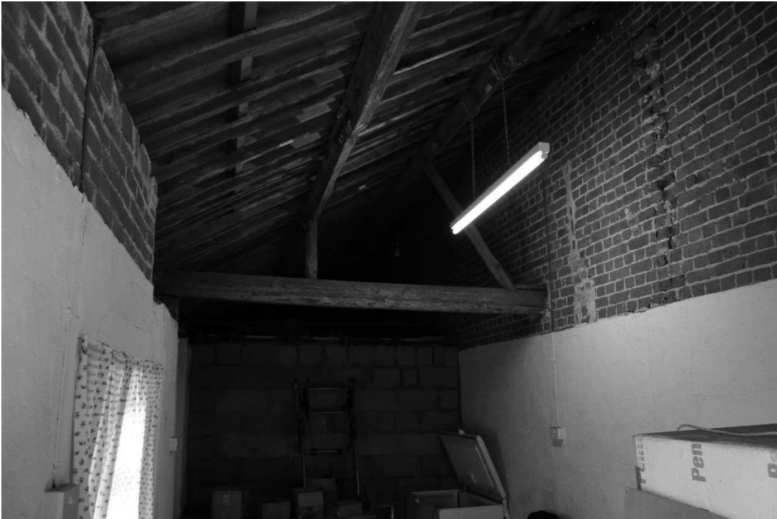
14. Rear offshoot roof looking towards right hand end
