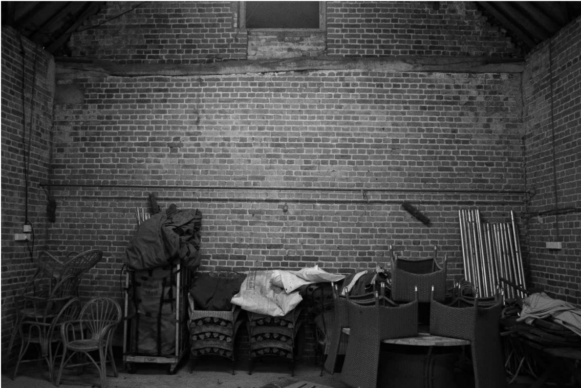
10. Internal view of left hand end wall
