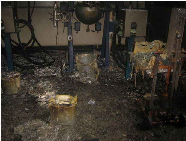
(Picture Identification: No 26 Internal Shot - Suspect seat of the fire).
